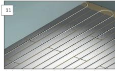
The heat distribution panels click into place in cleaned grooves. 17 mm water pipe are then installed.
