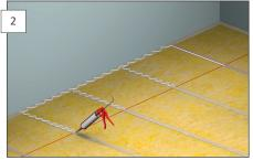
All free panel edges must be supported. If extra grooves for feed lines are to be cut out, extra support under the panels must be provided. The first row of panels is installed with the use of string. The panels must be glued to the subfloor or joists and fully glued at the tongue and groove. Recommended adhesive type is chipboard adhesive.
